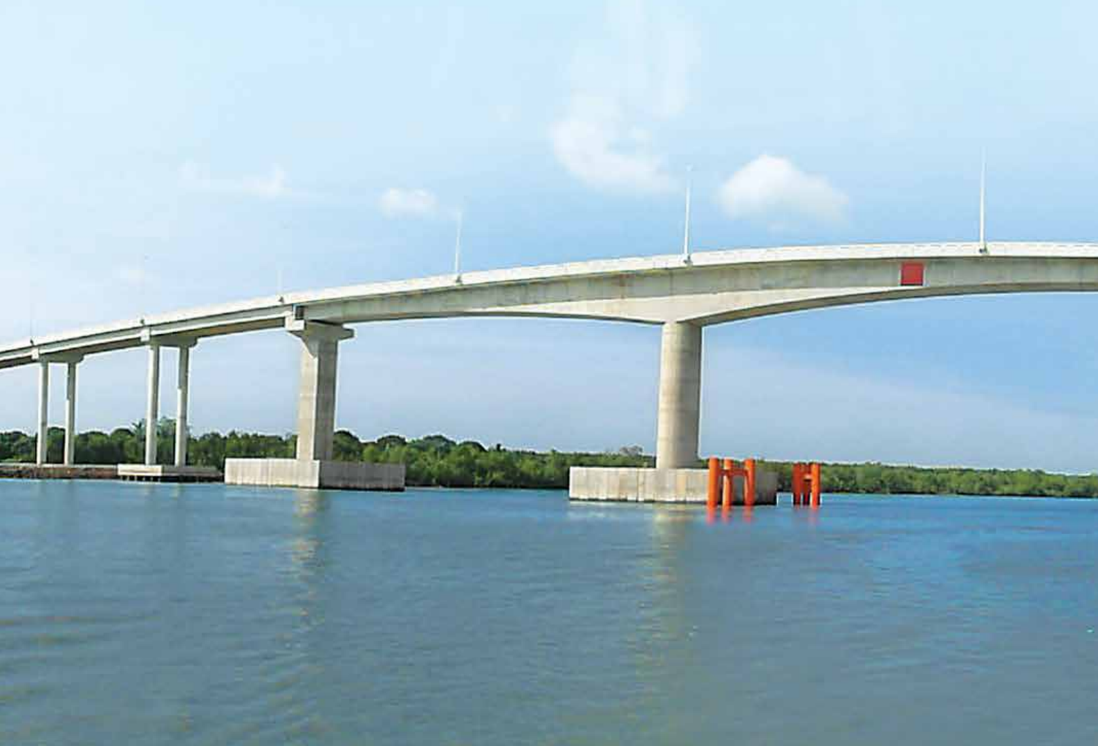
Bridge over Selat Lumut for South Klang Valley Expressway ("SKVE"), Selangor, Malaysia
