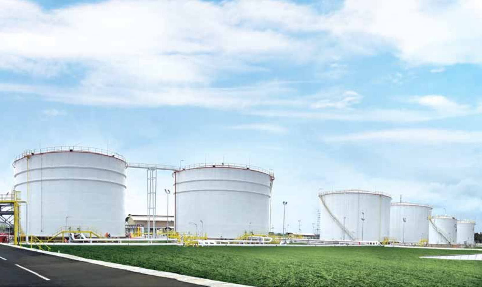
Engineering, Procurement and Construction of Central Oil Distribution Terminal (“CODT”) in Tanjung Manis, Sarawak, Malaysia
