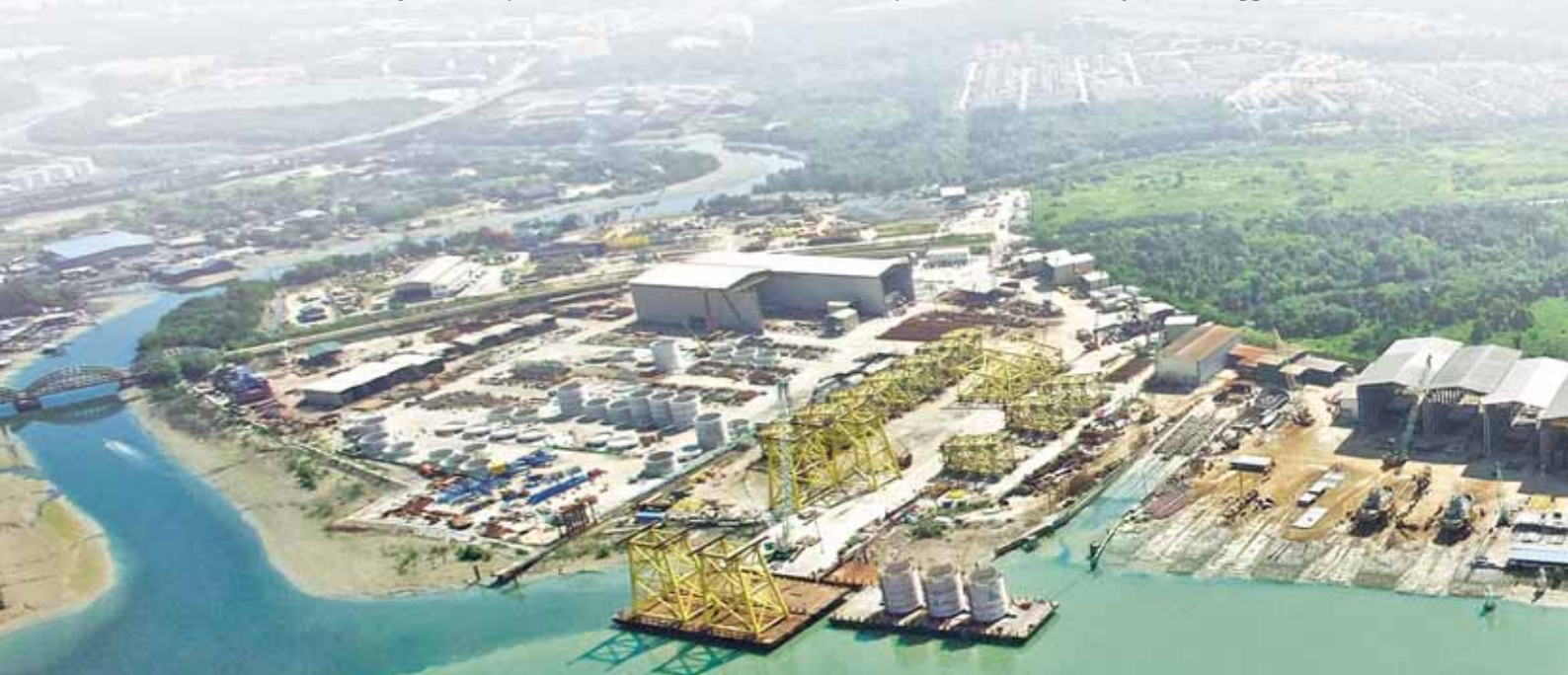
Fabrication yard of Muhibbah Steel Industries Sdn Bhd at Telok Gong, Port Klang, Malaysia
