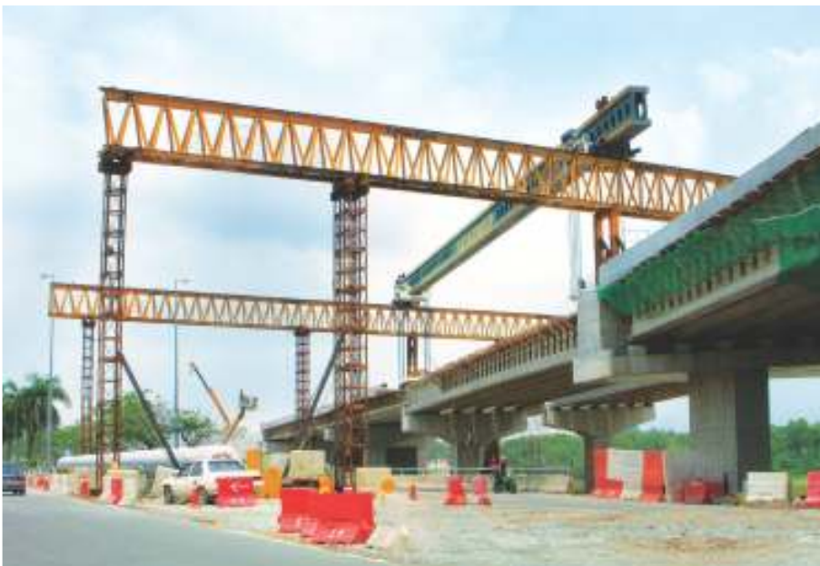
Bridge launching and Bridge foundation construction in progress for South Klang Valley Expressway ("SKVE") Project, Malaysia
