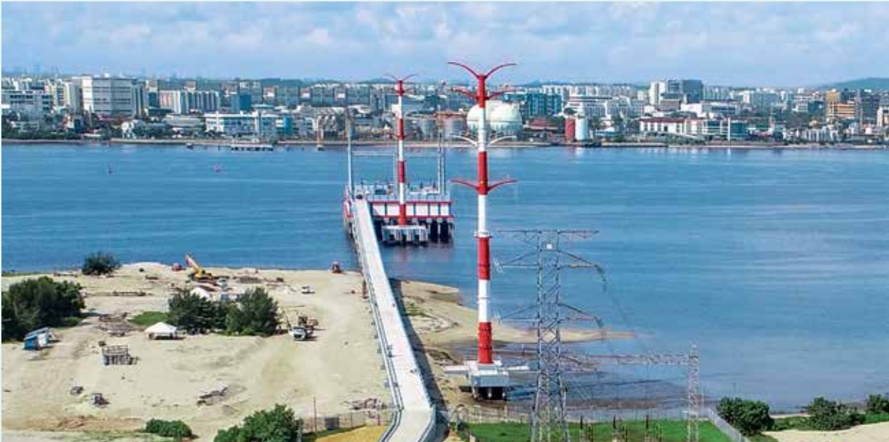
230kV TNB Senibong Switching Station Overhead Line, Johor Bahru, Johor
