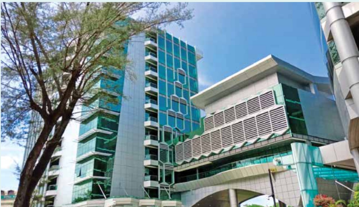
11-storey new office building complete with 2½ floor sub basement and car park at Kota Kinabalu, Sabah
