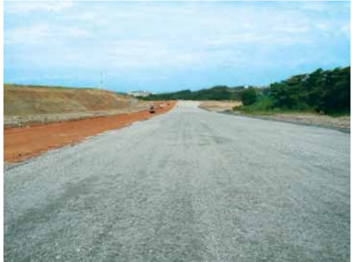
Road base work in progress for SKVE Project
