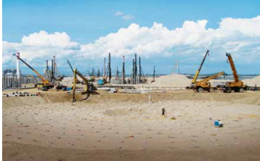
Tank Foundation work at Asia Petroleum Hub Project in Johor
