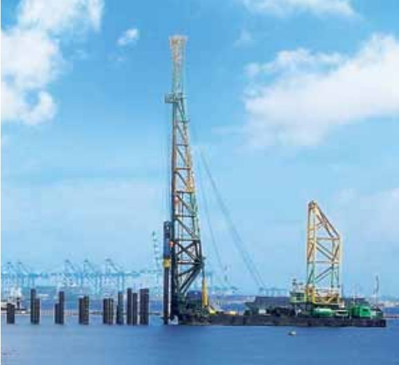
Jetty Works of Asia Petroleum Hub Project in Johor
