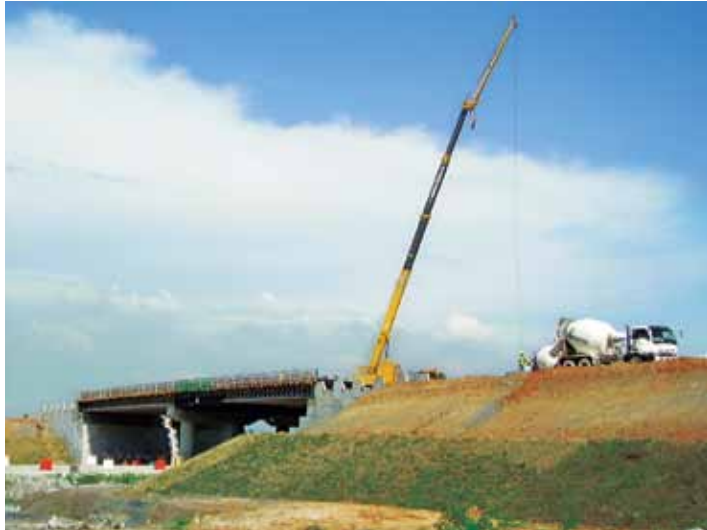
Bridge work in progress for SKVE Project
