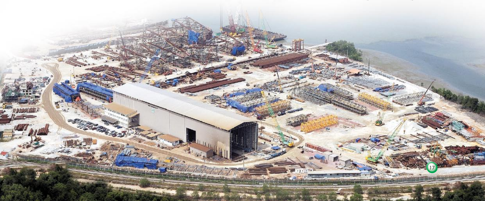
Fabrication Yard of Muhibbah Steel Industries Sdn Bhd
