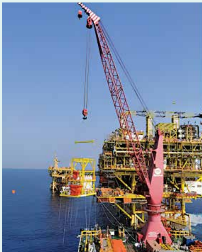
Acid Gas Removal Unit (AGRU) at Yetagun
