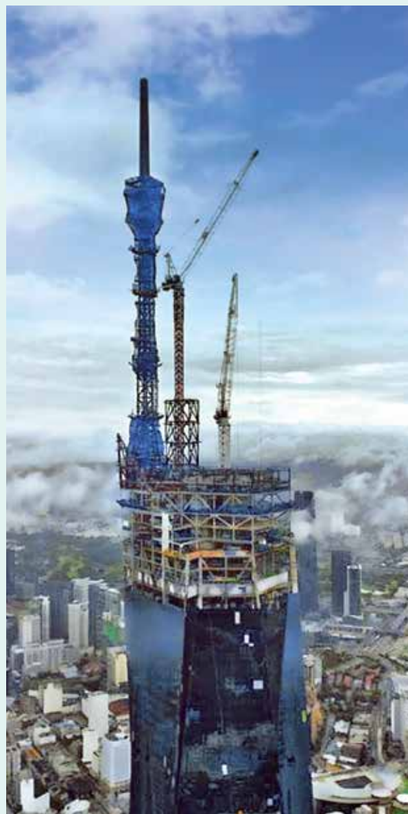
Favco Tower Crane for construction of PNB 118 Tower in Malaysia
