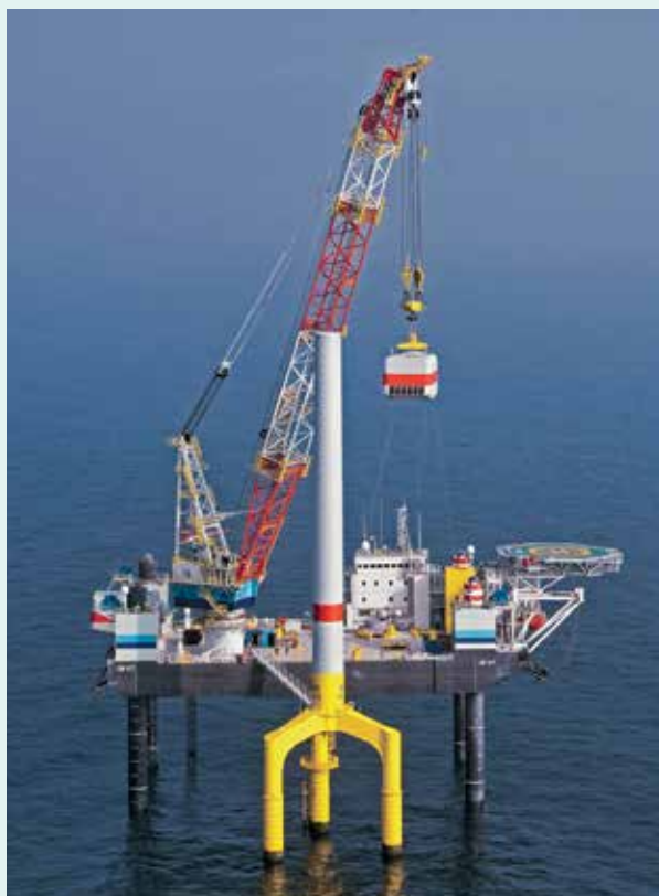
Favco offshore crane to install offshore wind turbine in Danish Waters
